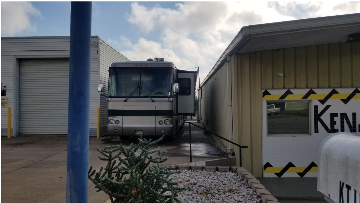
South area of the existing building to be expanded for an 18-wheeler service bay
